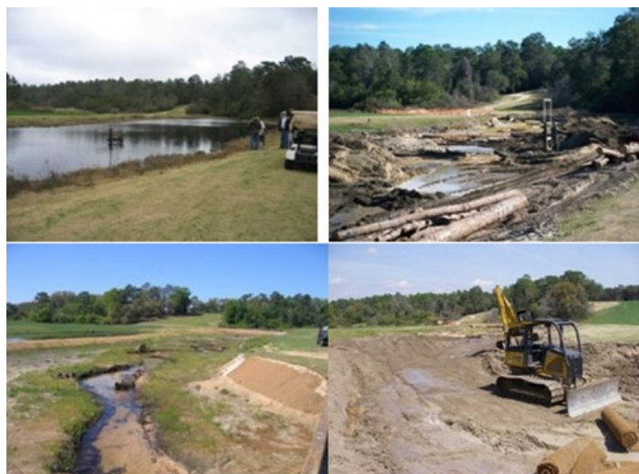
The process of restoring an Okaloosa darter stream on the Eglin Golf Course, clockwise from top left. A pond is drained and excavated so the floodplain can be rebuilt before the stream is created. Okaloosa darters colonized the new habitat within three months.
