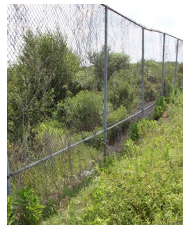
Airfield fencing in 2015 at Joint Base McGuire-Dix-Lakehurst (JBMDL) before replacement
