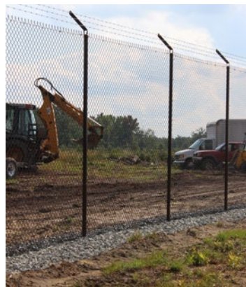
Airfield fencing in 2018 at Joint Base McGuire-Dix-Lakehurst (JBMDL) after replacement
