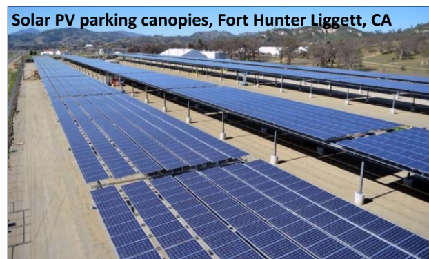
Photo: U.S. Army Corps of Engineers
